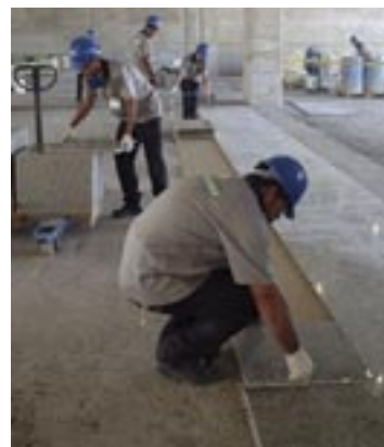
Processo na 3ª fiada In the third row, during the process
